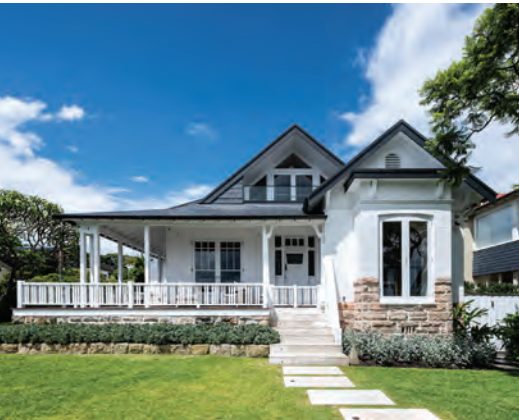
Project: Wolseley Road House
